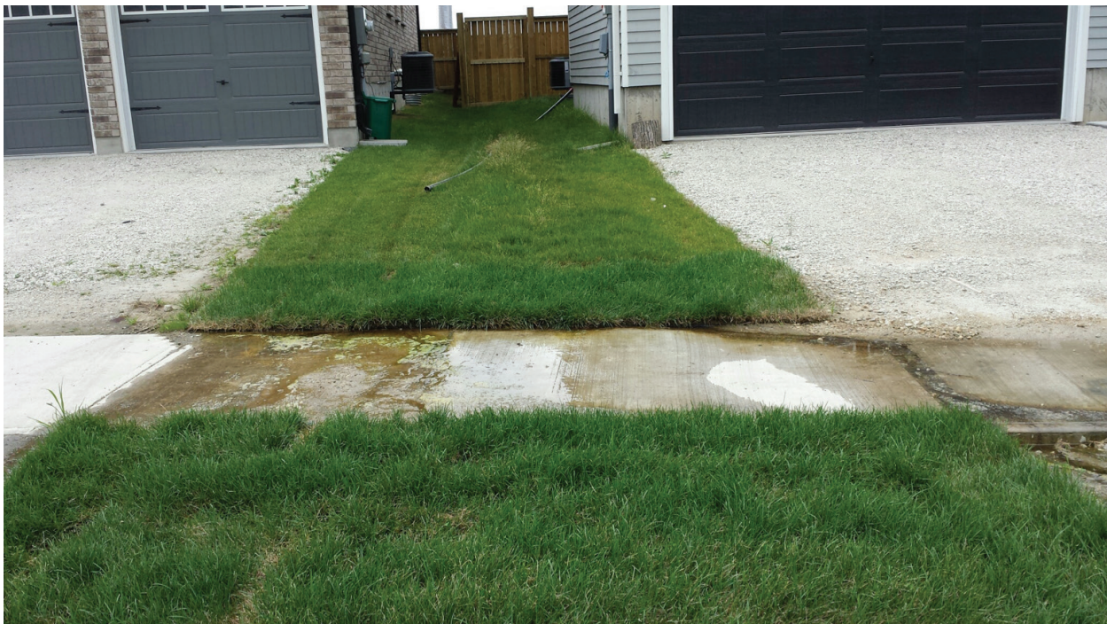
Figure 3b: Saturated Yard Resulting from Sump Pump Discharge (Collingwood, Ontario) 39
