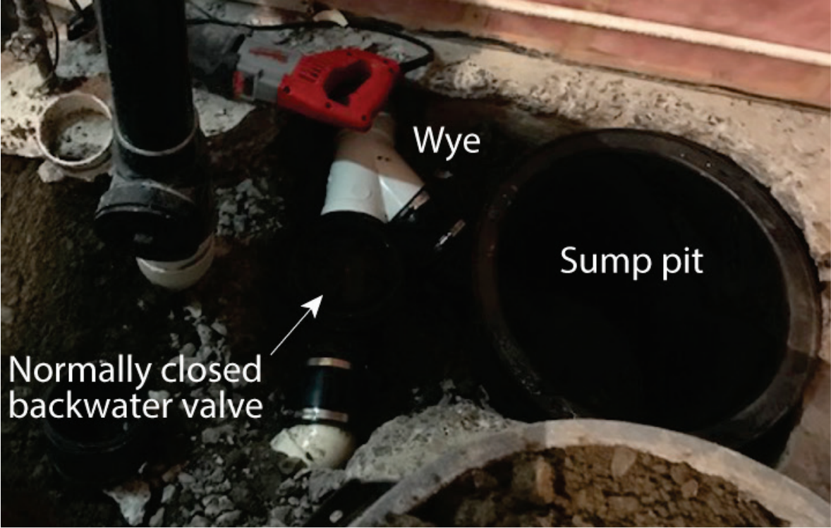
Figure 3h: Sump Pit and Backwater Valve Combination (Ottawa, Ontario) 49
